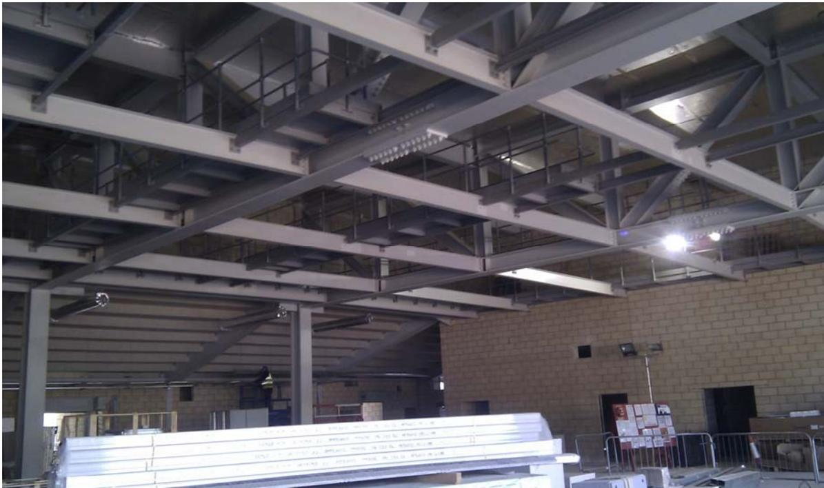
Figure 3: Conference Hall under Construction – Internal AHU Mounted in Gantry Area
