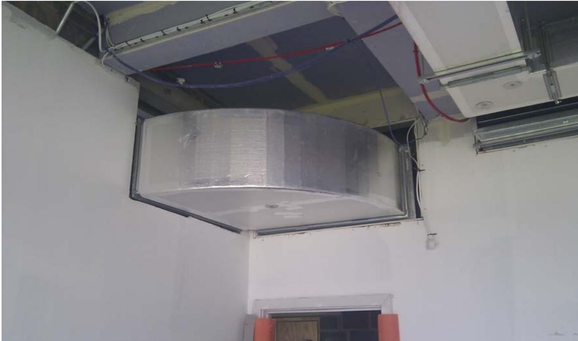
Figure 2: Due to spatial requirements the duct from the In-Vision Studio had to run through the adjacent TV studio and required careful independent boxing out
