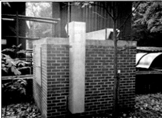
Figure 4, The 'Brick out-house', a ventilated acoustic enclosure for a centrifugal pump.
